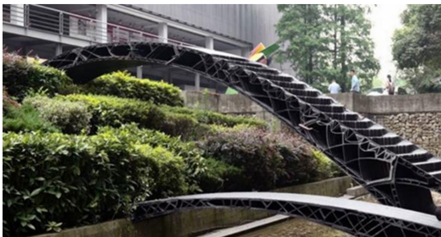
Fig. 2. A pedestrian bridge made of plastic in the 3D print technology, where the span measures 11 meters
